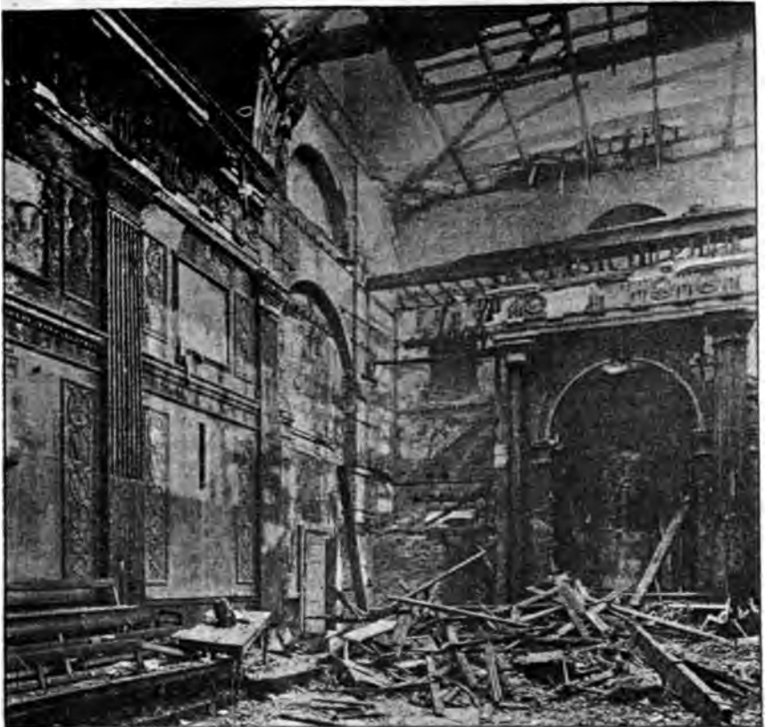
SOUTH END OF FREEMASONS' HALL, AFTER FIRE OF MAY, 1883.
